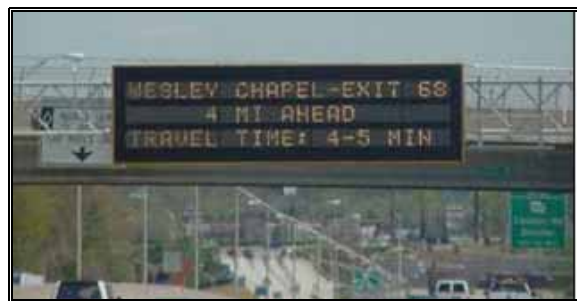
Figure 9: DMS Travel Time Message in Atlanta, GA (Source: http://www.georgia-navigator.com/about )
