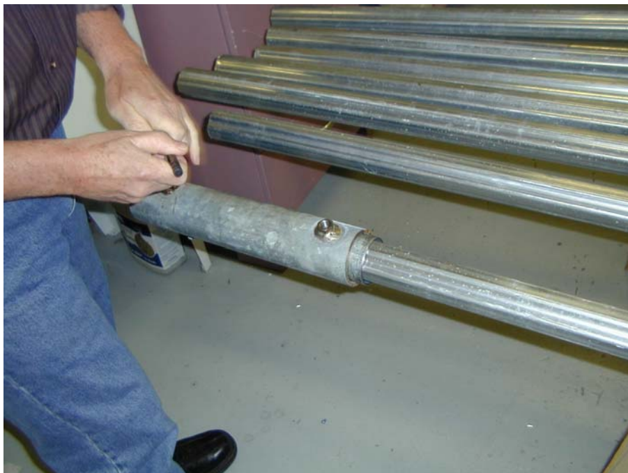
Figure 3: Adaptor to Fit the NexPole to Existing Sleeve
